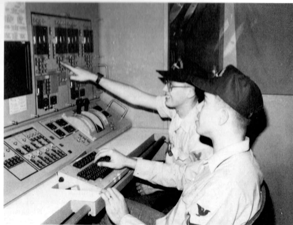
DDG-51 pre-commissioning crew members, GSE2 Joseph M. Doliana (left) and GSE2 Aaron P. Hunt, start a gas turbine engine at the PACC console on the site.
